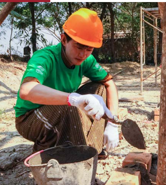
項明生認真砌磚 James Hong builds the foundation
